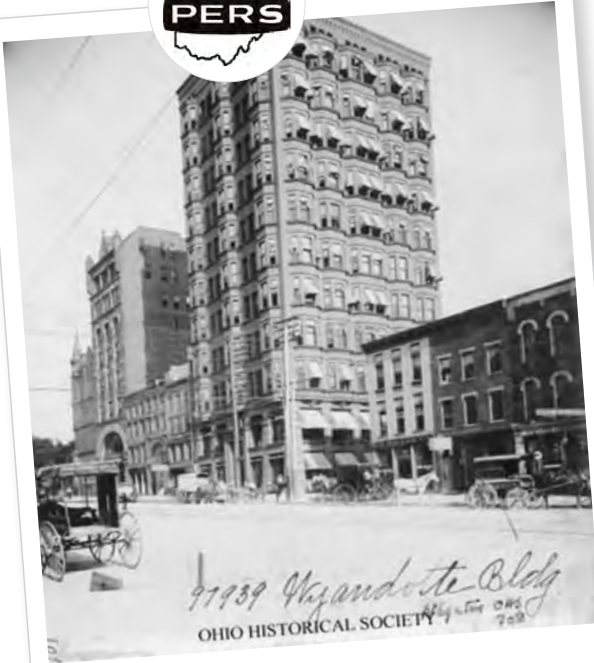
97939 Wyandotte Bldg OHIO HISTORICAL SOCIETY APR 19 1908 Wyandot Building, home of PERS until 1937.
