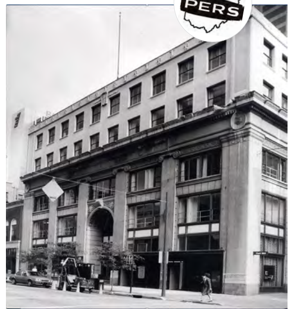
Nitschke Building, home of PERS from 1937 to 1970.
